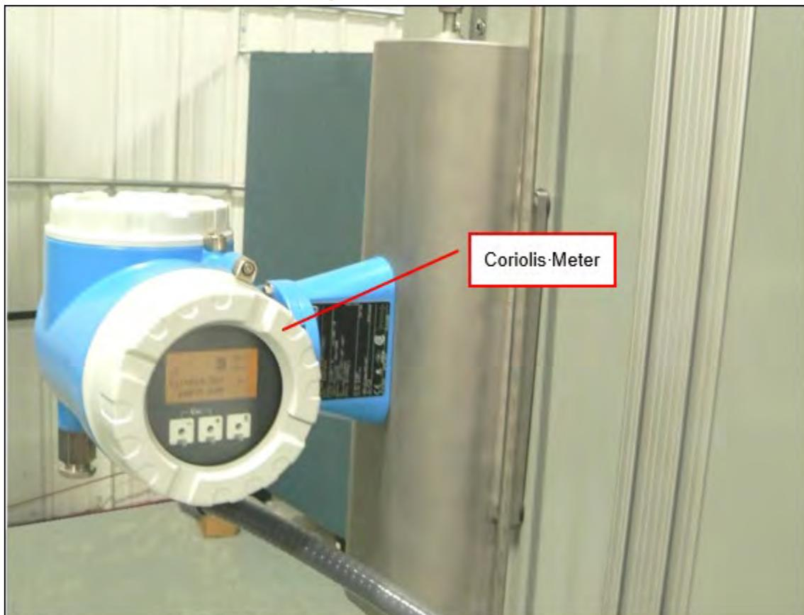
*Figure 10: Fuel Flow Measurement and Fuel Conditioning Components*
