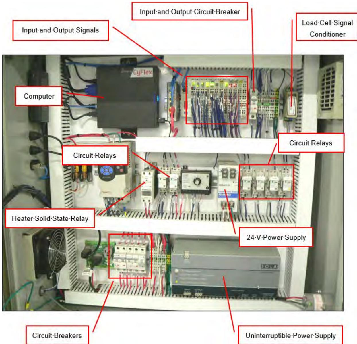
*Figure 6: Circuit Breakers – Bottom Rack*
